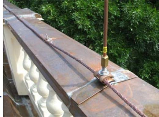
In this installation, air terminals are secured to copper straps which are soldered to the new copper balustrade cap, providing a strong connection without puncturing the cap with mechanical fasteners. ▶
