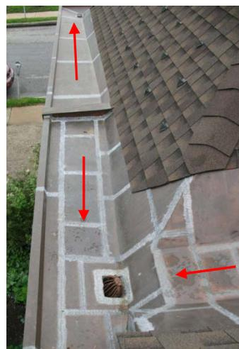
Figure 1: Built-in gutter and gusset intersection
