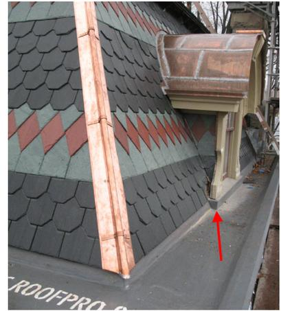
Figure 2: Dormer window sills within the built-in gutter. ▶
