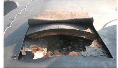
▲ Single layer of polyisocyanurate insulation. The insulation warped as a result of condensation on its underside and fastener corrosion. Source of the moisture – interior air.
