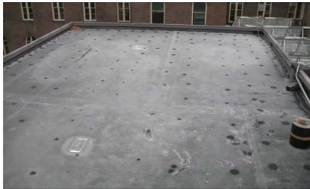
◀ The dark round circles in this photo indicated the insulation’s fastener pattern. The fastener plates are frost-free due to thermal bridging. It is estimated that thermal bridging of fasteners reduces the R-value of insulation by 8 to 10 percent.
