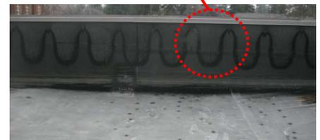
▲ Frost patterns on the EPDM clad parapet walls formed a perfect sine wave. The distance between the peaks of the non-frosted areas matched the width of the insulated metal wall panels exactly, confirming our earlier observation of air movement from the interior into the roof system, but also vividly showing the degree of heat loss through the joints between panels.
