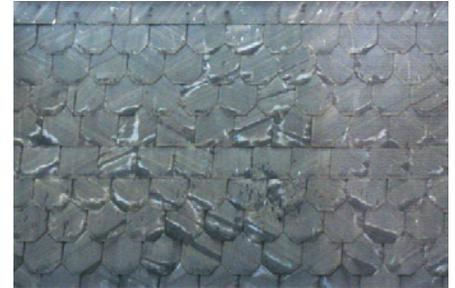
After some years of exposure, hard-vein slate used for roofing purposes takes on a more pronounced streaked appearance as the ribbons become more prominent and can be seen to be oriented at various, random angles across the face of the slate (see photo at bottom of column). In some environments, weathered slates can take on a light orange hue. Wall cladding slates sometimes turn a matte green color.
