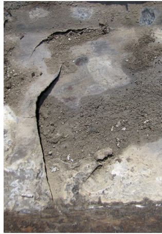
Fatigue cracks in a flat seam gutter formed from large pans with no expansion joints.
